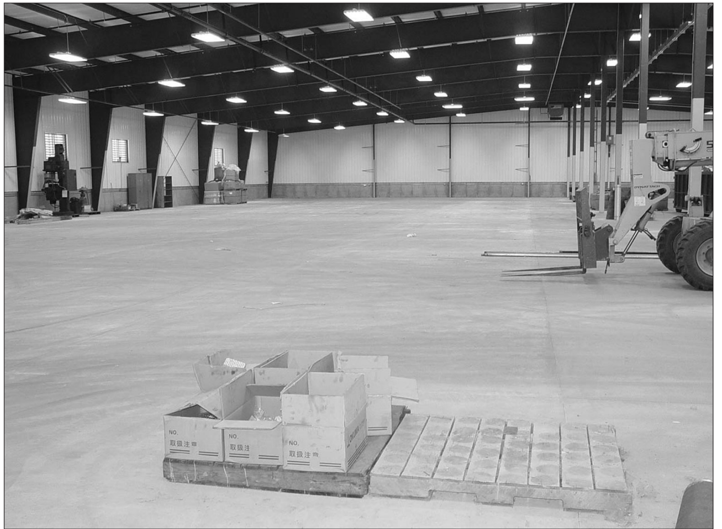
The construction of the 41,000-square-foot addition (Building #39) on the south side of the plant is completed.
