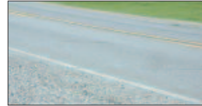
Resurfacing shoulders on Hwy. 34
